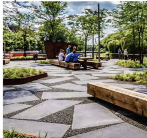
SPECIALTY SEATING & SALVAGED CONCRETE PAVING
