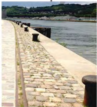
COBBLE PAVING & LIGHTED MARKER
